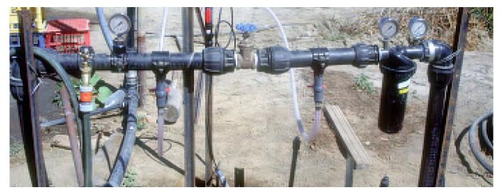
A simple manifold set up with a venturi injector, pressure gauges and a valve causing the required pressure drop.
