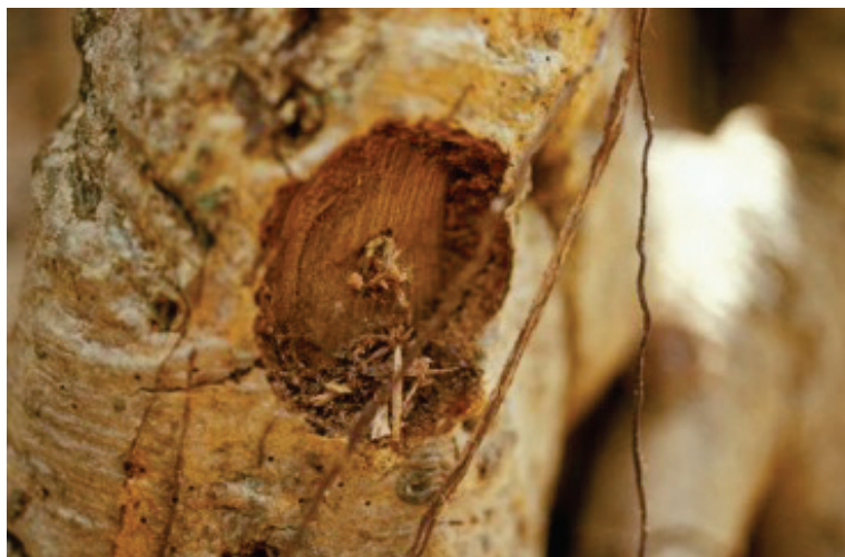
Figure 4. Damage to the trunk with the entrance plugged up with frass
