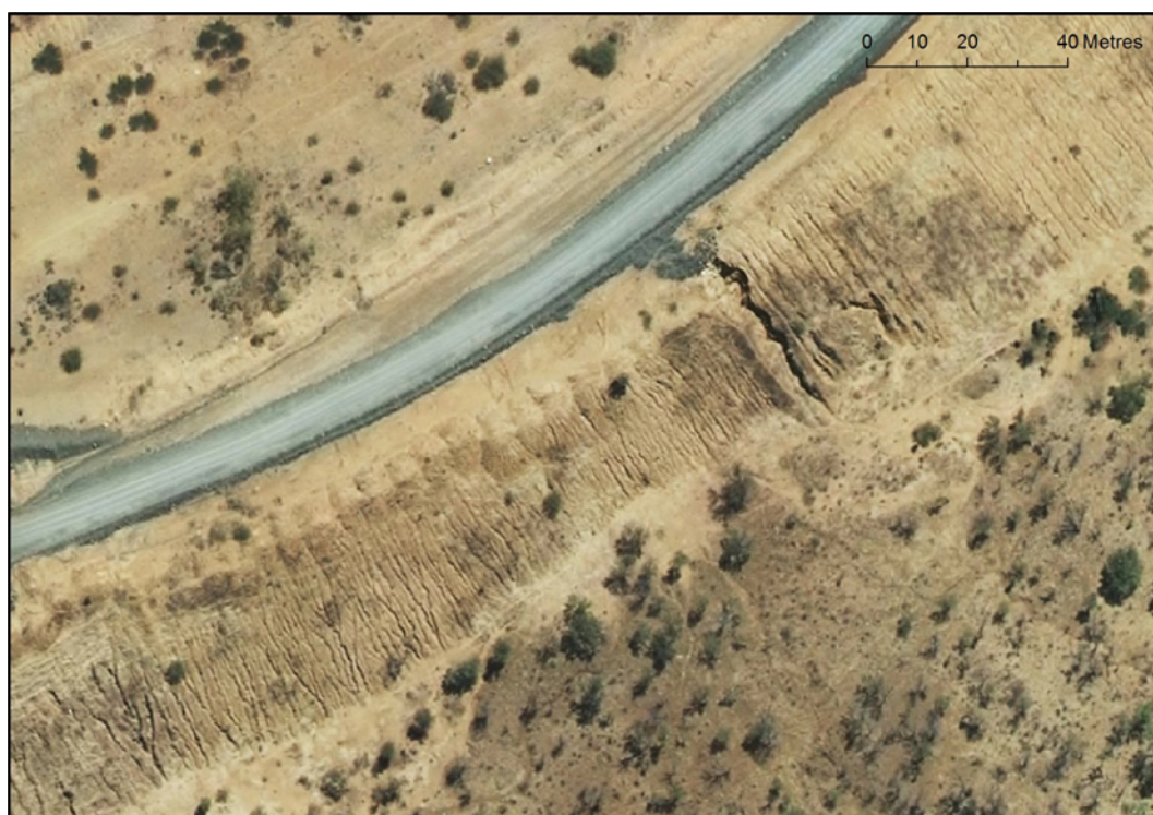
Plate 4.2 – Erosion into the Mine Levee Wall at Location 2 (see Figure 4.7)
