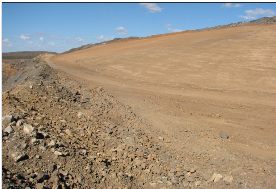
Plate 4.6 – Paddock Dumping and Roller Compaction of PAF(HC) and PAF(RE) on Northern Part of NOEF
