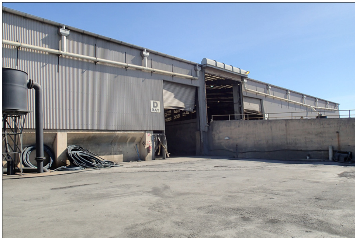
Plate 4.25 – Open Doors on the Concentrate Shed and Visible Concentrate Dust at the Bing Bong Loading Facility
