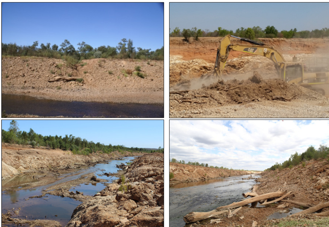
Clockwise from top left: 1) Typical lower diversion river bank in 2013. 2) Burying LWD. 3) and 4) Lower diversion during on-site visit by IM in June 2015. Note the captured sediment, which has tubestock planted in it; and the diversion immediately post-LWD installation.
