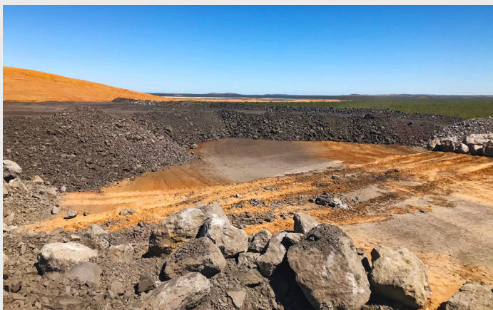
2-m Dumped PAF Rock Ready for Compaction
