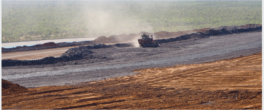
Bulldozing PAF Cell - NOEF
