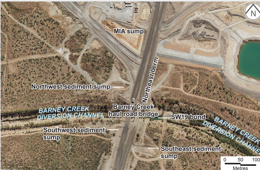
Sediment Control Structures Near Barney Creek Haul Road Bridge
