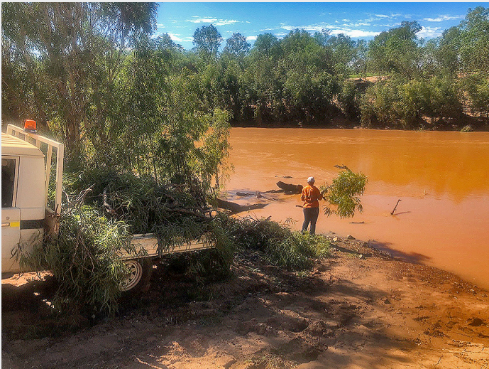
Small Woody Debris Being Placed into the McArthur River Diversion Channel
