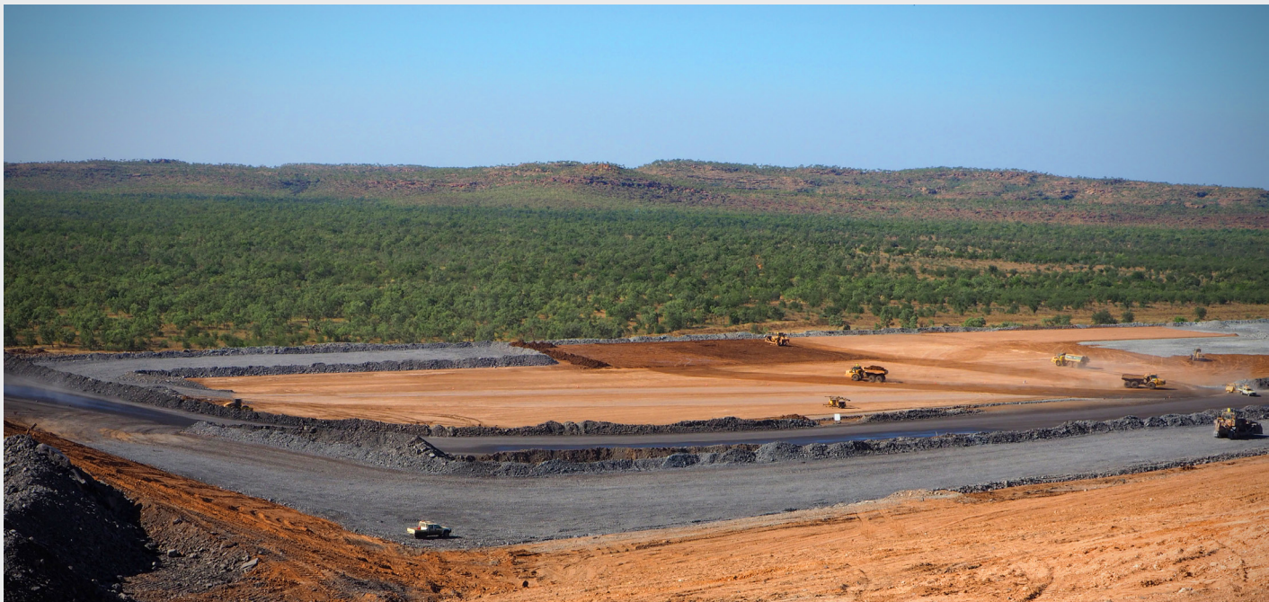
Construction Activities on Central West Stage of the NOEF
