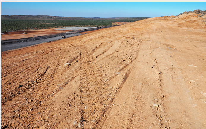
Interim Barrier to Help Prevent Transfer of Heat Between Older Dump Area and New Central West Stage
