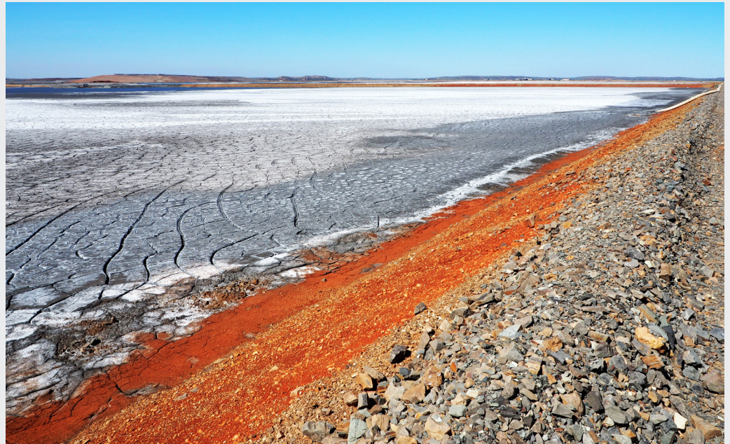
Salt Crusting on the Surface of TSF Cell 2
