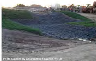
Photo 1 – Rock mattress lined basin spillway and energy dissipater
