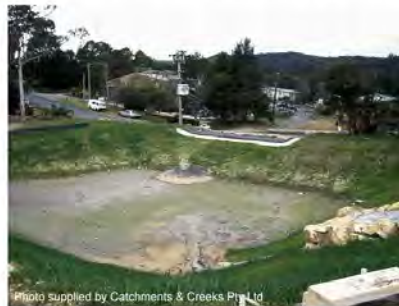
Photo 18 – Rock-lined spillway—note concrete sealing of the spillway crest
