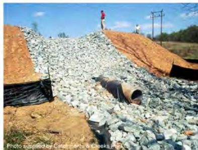
Photo 1 – Rock-lined sediment basin spillway with low-flow pipe outlet
