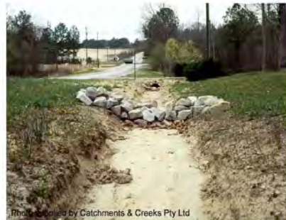
Photo 2 – Rock check dam
