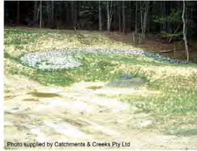
Photo 16 – Emergency spillway located within virgin soil to the side of the embankment
