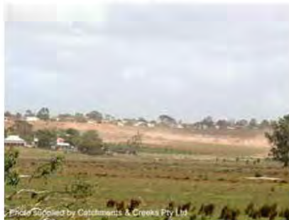
Photo 1 – Dust generation on a construction site
