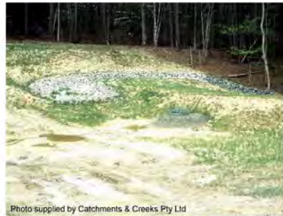
Photo 4 – Rock-lined spillway cut into virgin soil (note the spillway is curved up to the crest, after which it remains straight)
