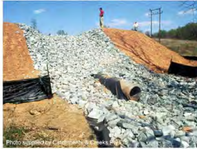
Photo 15 – Emergency spillway located within the fill embankment
