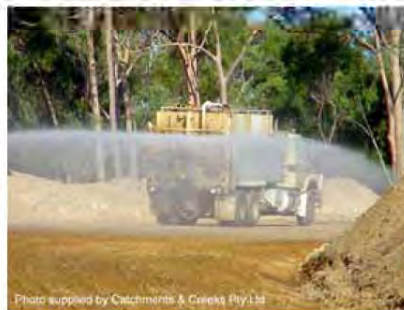
Photo 2 – Dust control using a water truck
