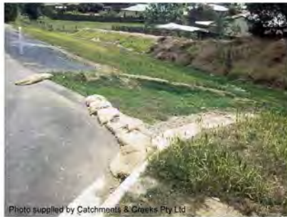
Photo 3 – Sandbags (temporary) used to control flow entry into grass chute
