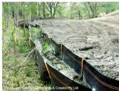
Photo 8 – Double sediment fence
