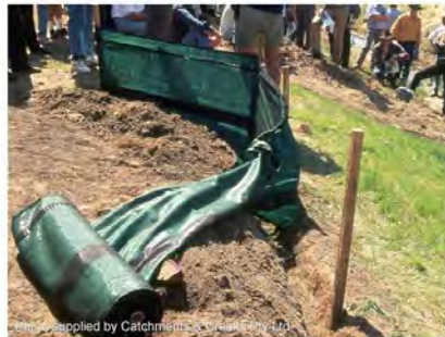
Photo 1 – Installation of a sediment fence
