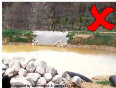
Photo 7 – Spillways must have a well-defined profile to fully contain the flow
