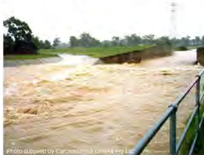
Photo 6 – Hydraulic jump dissipater downstream of detention basin outlet
