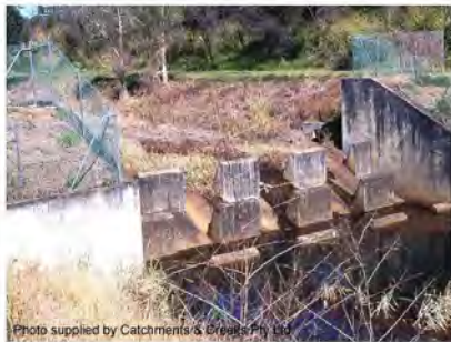
Photo 11 – Baffled spillway
