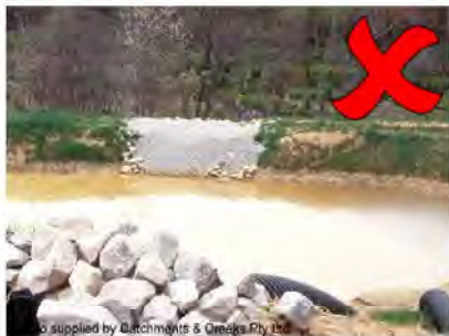
Photo 13 – Spillways must have a well-defined profile to fully contain the flow
