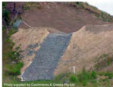
Photo 2 – Rock mattress-lined sediment basin emergency spillway
