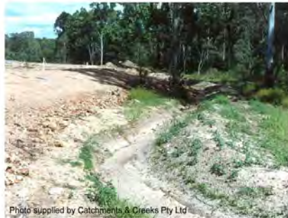
Photo 1 – Temporary diversion channel collecting 'dirty' water down-slope of a soil disturbance
