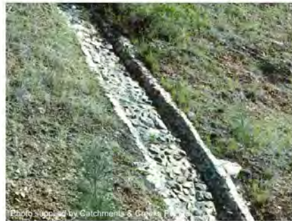
Photo 1 – Permanent, grouted-stone batter chute
