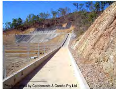
Photo 2 – Permanent diversion channel collecting stormwater runoff up-slope of a subdivision
