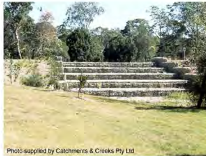
Photo 3 – Permanent, gabion-lined stepped spillway located on a detention basin
