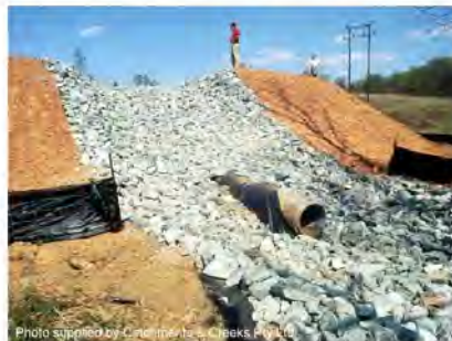
Photo 5 – Hydraulic jump type energy dissipater on sediment basin spillway
