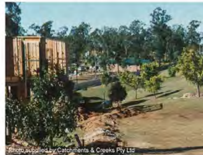
Photo 2 – Flow diversion bank up-slope of a building site
