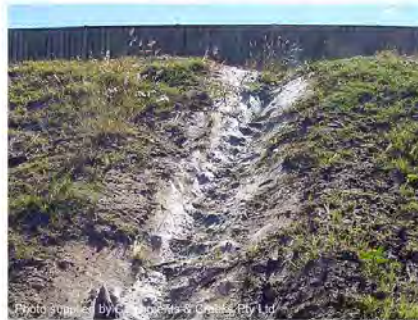
Photo 2 – Temporary batter chute lined with filter cloth
