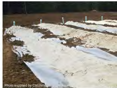
Photo 14 – Sand filter outlet system during installation
