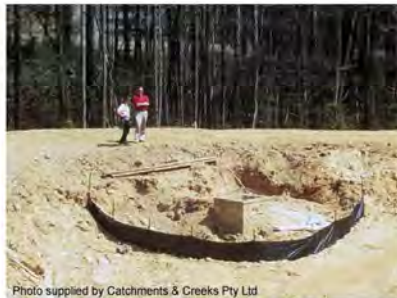
Photo 5 – Outlet chamber
