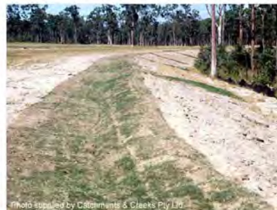
Photo 6 – Turf-lined flow diversion bank with grass-lined outlet chutes at regular intervals along the embankment
