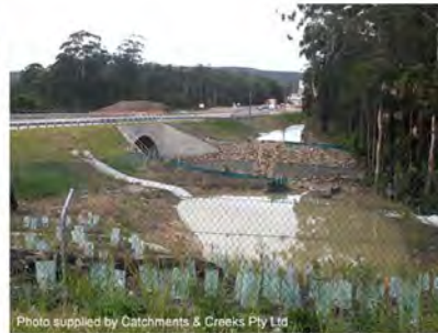
Photo 24 – Sediment basins converted to permanent stormwater treatment ponds on highway project
