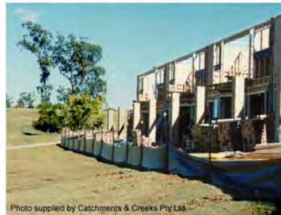
Photo 2 – Sediment fence located down-slope of multi-dwelling building site
