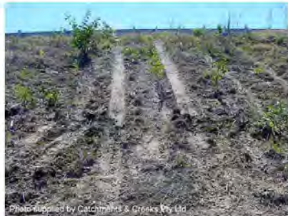
Photo 5 – Wheel track marks down a slope potentially causing concentrated runoff
