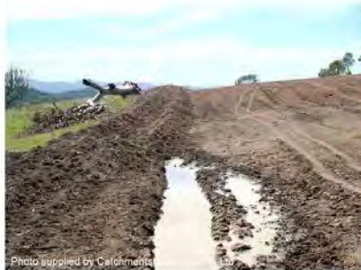
Photo 1 – Flow diversion bank down-slope of a future pipeline installation
