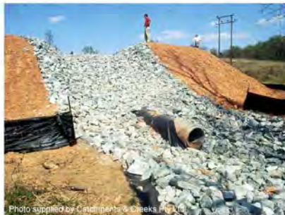
Photo 5 – Spillway chute with well-defined inlet profile
