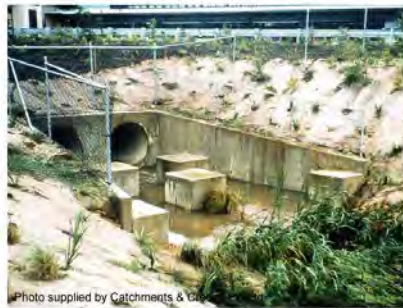
Photo 12 – Impact block energy dissipater
