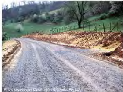
Photo 1 – Gravelling of construction access road
