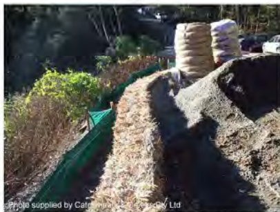
Photo 7 – Use of straw bales to prevent direct contact of stockpiles with the fence
