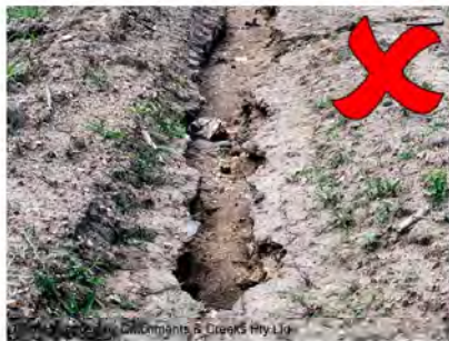
Photo 5 – Upper limit of erosion within a catch drain
