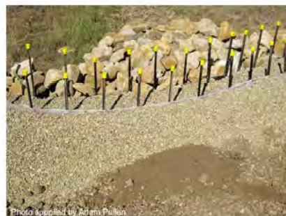
Photo 6 – Upstream face of a sediment weir
