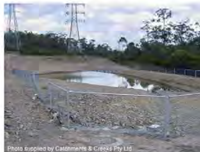
Photo 22 – Temporary fencing of a construction site sediment basin
