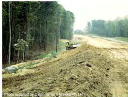
Photo 1 – Tracked vehicle walking up and down slope
