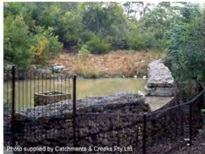
Photo 23 – Permanent sediment basin within residential estate
