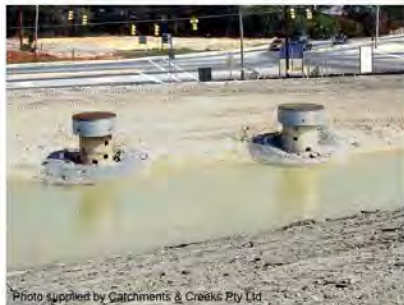
Photo 9 – Twin riser pipes in the process of being installed
