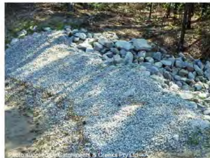
Photo 4 – Rock filter dam with aggregate filter
