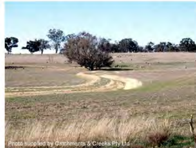
Photo 2 – Large rural catch drain (channel-bank)
