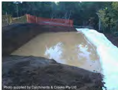
Photo 17 – Fully recessed basin with natural ground forming the spillway
