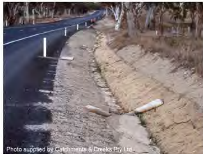
Photo 1 – Sandbag check dams
