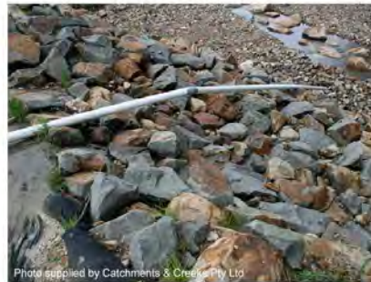
Photo 6 – Spillways lined with loose rock generally have a high risk of failure compared to concrete and rock mattress linings
