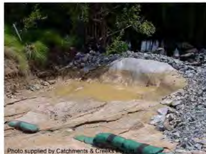
Photo 3 – Rock filter dam with geotextile filter
