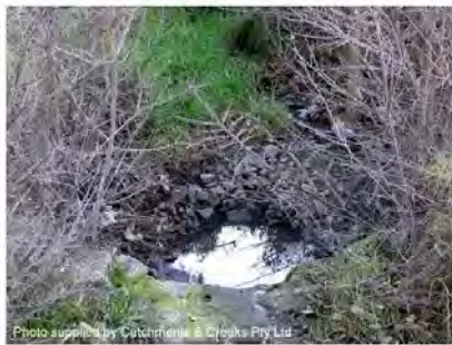
Photo 7 – Rock-lined plunge pool energy dissipater
