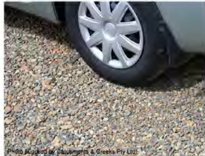
Photo 2 – Gravelling of construction site car park
