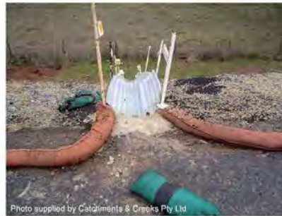
Photo 4 – Geotextile socks used to control flow entry into temporary batter chute
