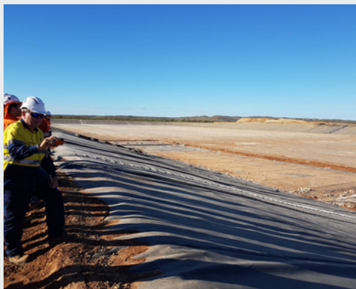
Western PAF runoff dam
