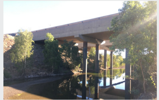
Barney Creek haul road bridge
