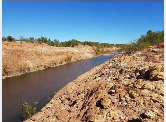
Middle to downstream section of the diversion channel showing extensive erosion of banks
