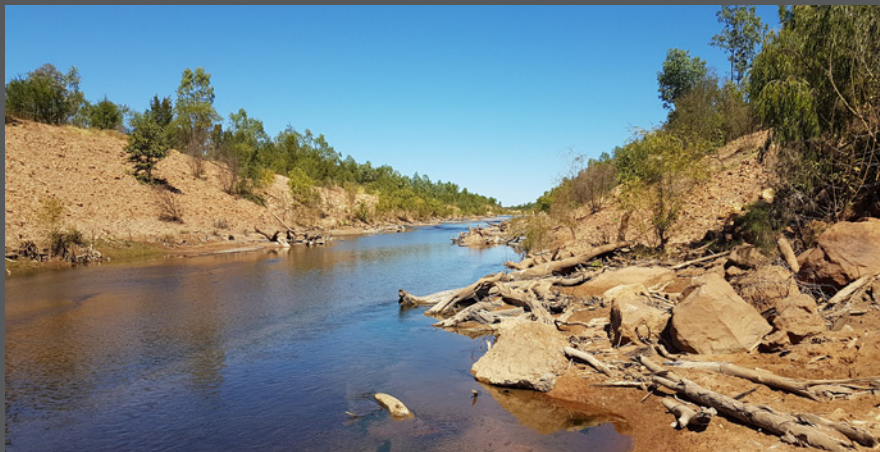
McArthur River diversion channel
