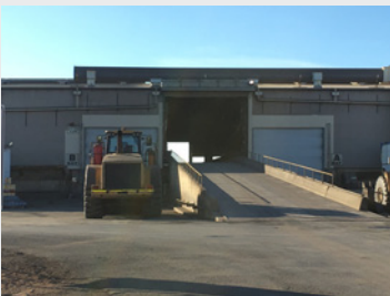
New smaller roller doors of the concentrate storage shed
