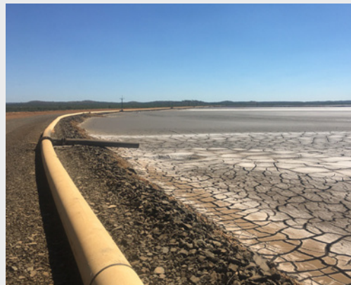
TSF Cell 2, showing tailings pipeline
