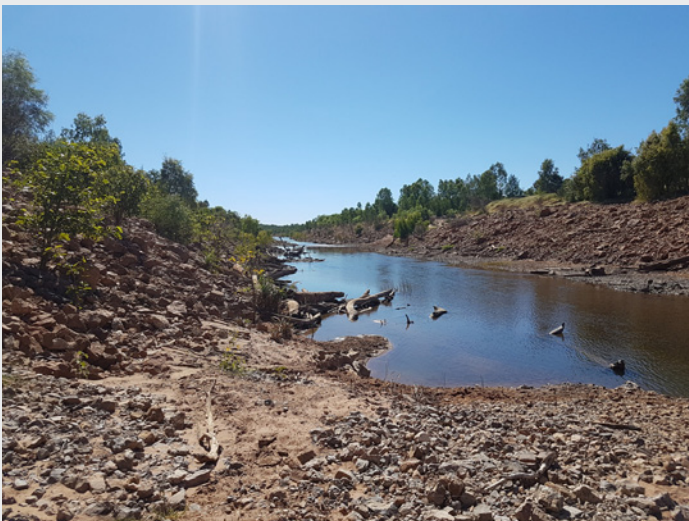
Downstream section of the diversion channel
