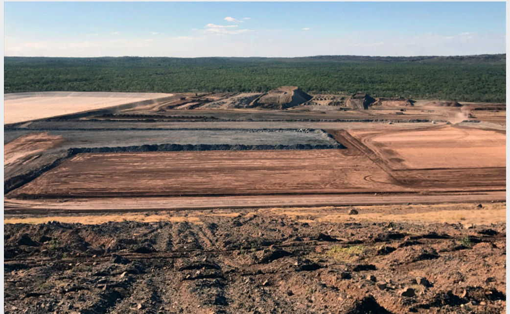
NOEF foundation preparations showing a compacted clay base followed by low salinity non acid forming waste rock
