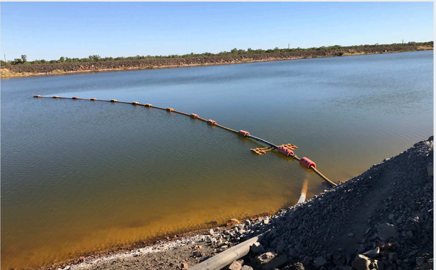
Seepage collected in the SPROD
