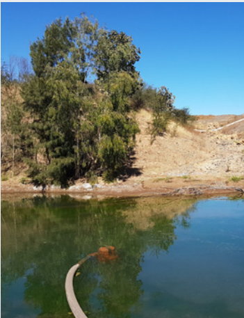
Dewatering pump located in downstream section of the Barney Creek diversion channel
