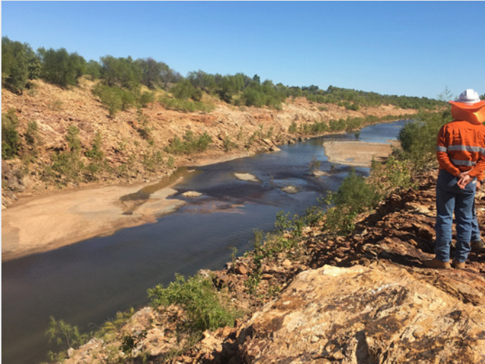
Revegetation in the middle to upper part of the McArthur River diversion channel
