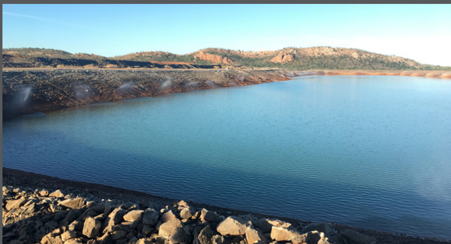
South east PAF runoff dam
