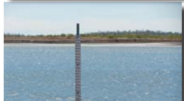
Top: Photo taken along the southern wall of TSF Cell 2 in May 2012. This wall will be raised to increase the capacity of Cell 2. Bottom: The level of water in Cell 2 at inspection is still of concern.
