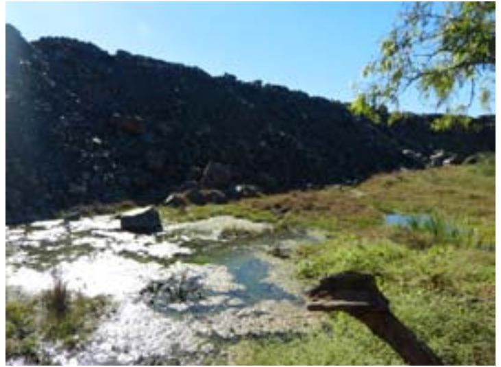
An area of seepage has been flowing from the north eastern toe of the Overburden Emplacement Facility.
