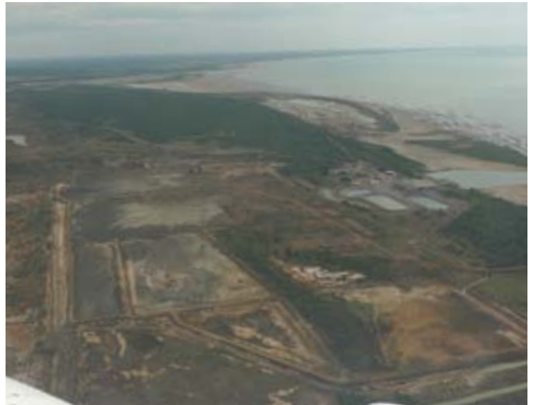
Aerial photograph of the Bing Bong port facility, which now has three surface water runoff ponds to contain contaminated runoff water.
