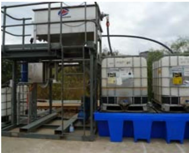
Groundwater treatment system used to recover diesel product from the impacted groundwater.
