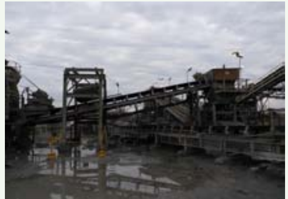
Dust suppression at the 'Pacrim' crushing plant has improved this audit period with the addition of sprays along the conveyor system. The IM noted a visual decrease in dust from this plant. Note the wet foreground from water sprays. Note though levels have come down, measured dust levels and lead is similar to previous years.
