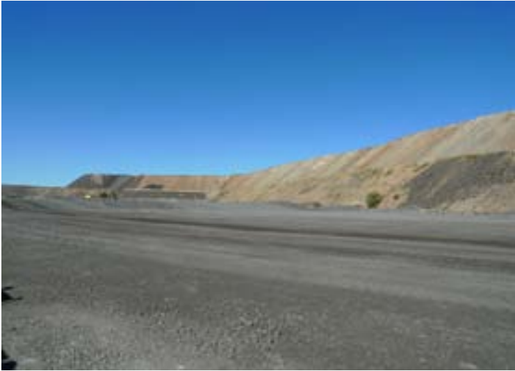
Waste rock placed in the Overburden Emplacement Facility (OEF) is potentially acid forming, and is placed strategically within the OEF according to design, to minimise the future potential for environmental damage.
