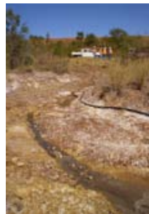
In May 2012, the seepage from the TSF Cell 1 appeared to be fresher than in previous years, as evidenced through the presence of algae and grasses along the drainage line.
