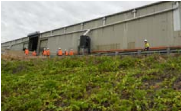
Water tanks have been installed around the Bing Bong concentrate storage shed to capture the first flush of rain water and divert consequent rainfall to sea, rather than to onsite storage
