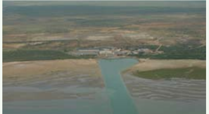
Aerial view of the Bing Bong swing basin, dredging channel and beach, May 2012.
