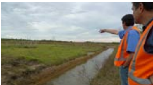
Members of the Independent Monitor team inspecting the Bing Bong diversion channel in May 2012.
