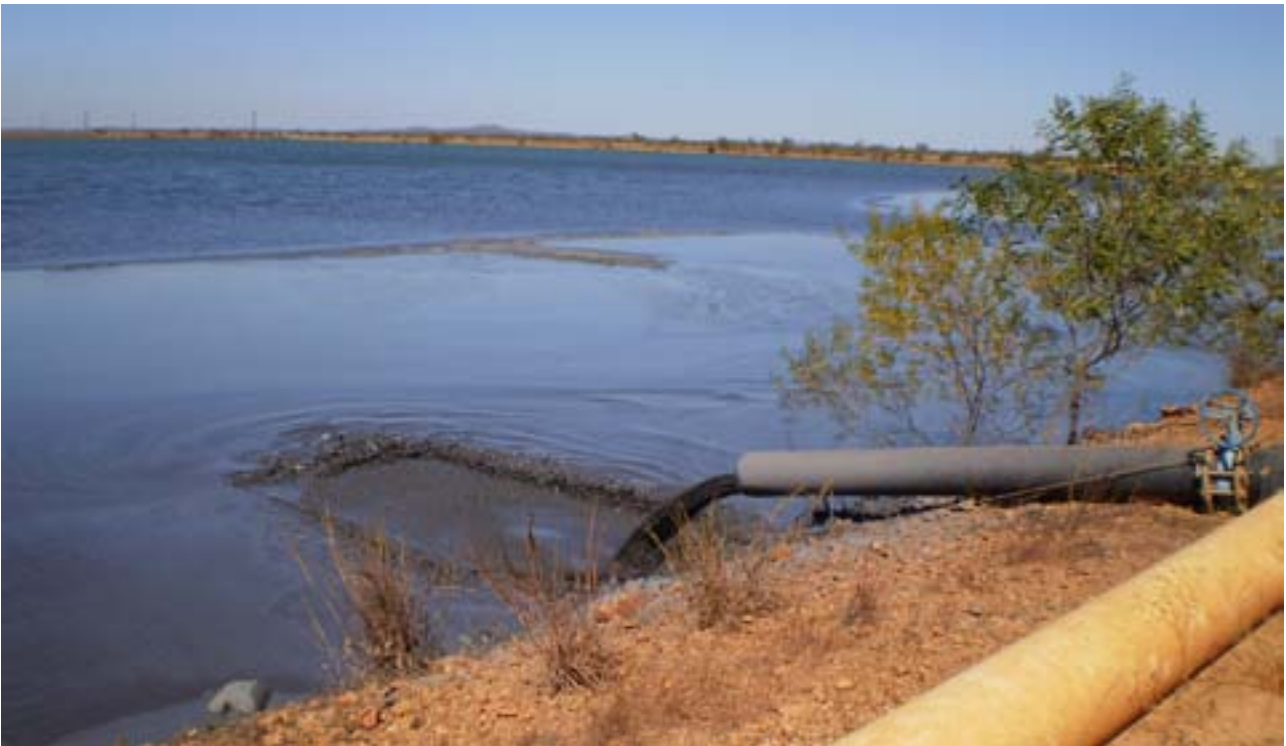
Aqueous deposition of tailings in TSF Cell2 observed by the IM during the May 2011 site inspection.
