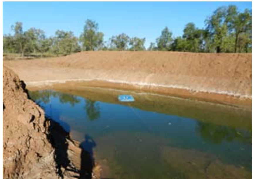
Seepage flowing from the toe of the OEF is collected in a sump and is pumped to an onsite containment dam - see previous page for details.
