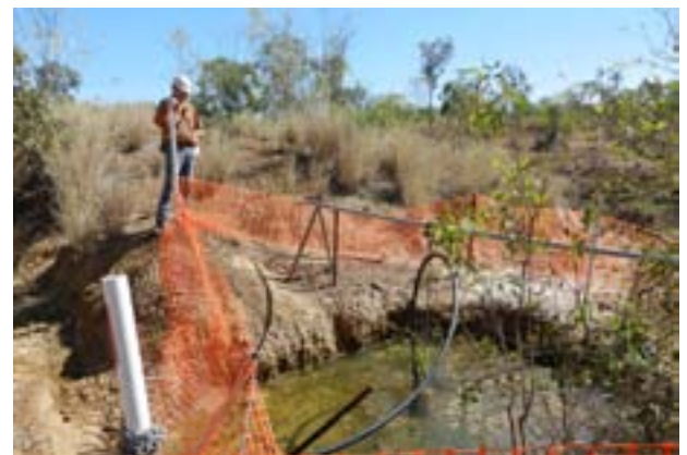
Seepage recovery sump between TSF Cell 2 and Surprise Creek, where a frog and macrophytes were observed. This indicates that the seepage water may be fresher than in previous years.
