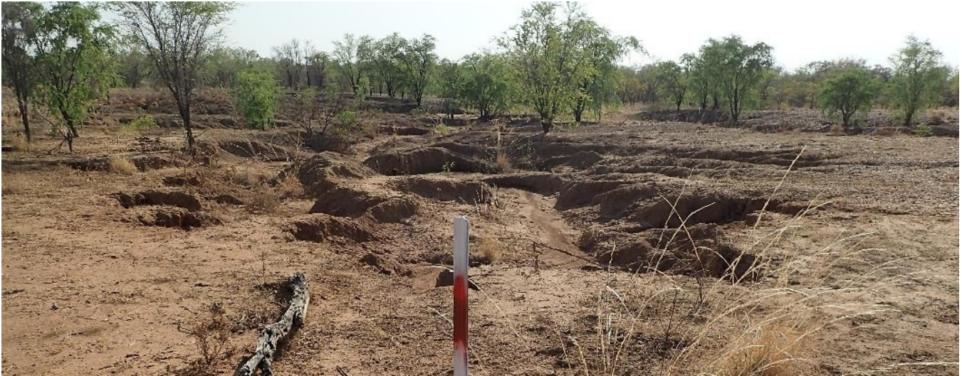
Figure 14. Sheet and gully erosion requiring management intervention. Photo: Caz Pettit DPIR
