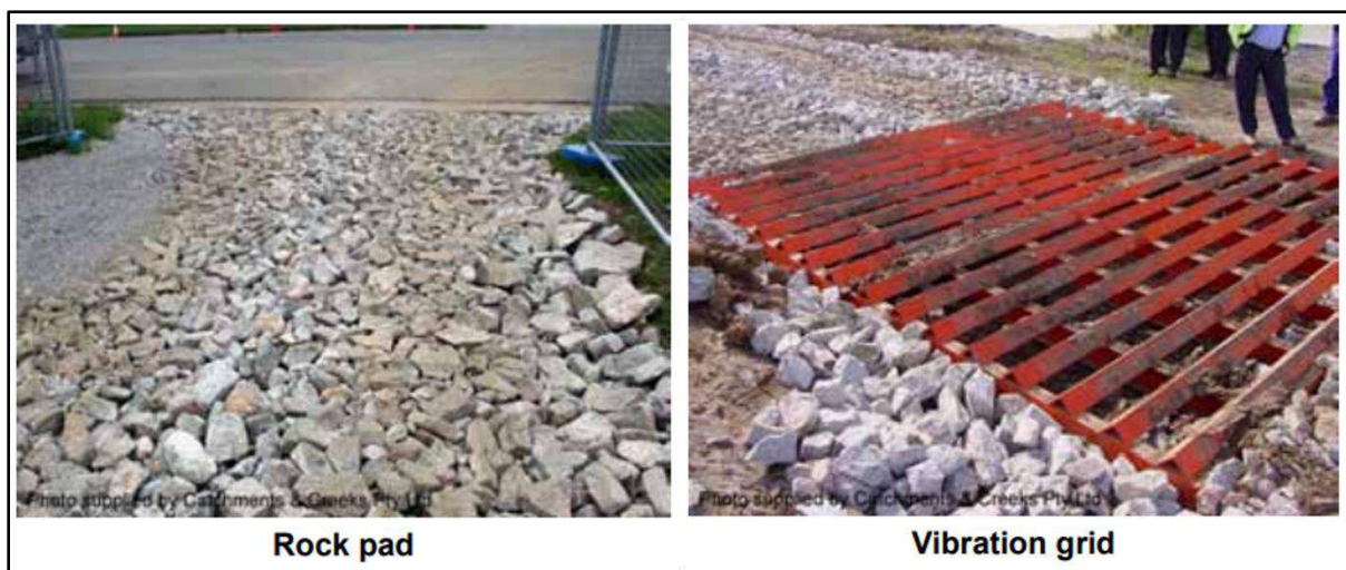
Figure 9 Example of Entry-Exit Shake Down Area (Source: Witheridge, 2012)
