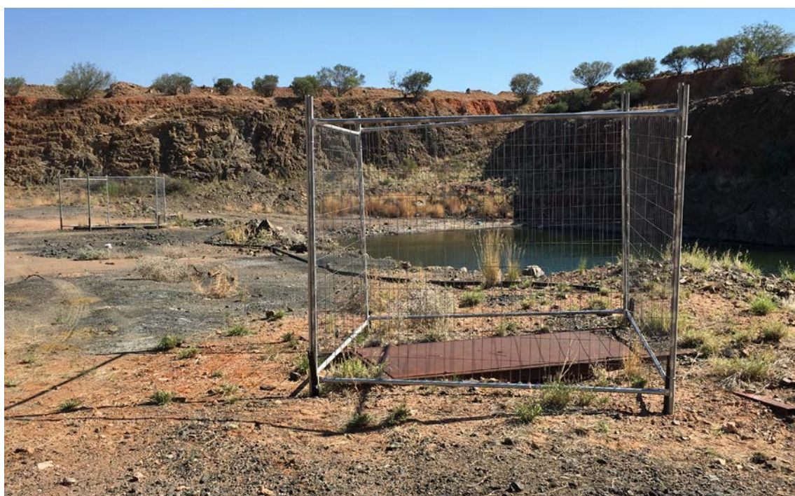
Figure 4: Barricading erected on two northern most bulk sample shafts in Molyhil pit.
