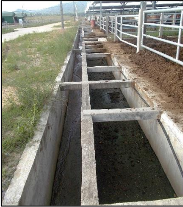
Figure 3.53: Suitable drainage for collecting effluent from holding yards.
