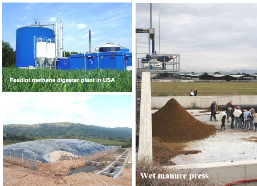
Figure 3.58: (Conterclockwise). Feedlot methane digester plants to generate electricity (USA and Vietnam); Manure press to separate liquid and solids from feedlot effluent for recycling as fertiliser (Italy).
