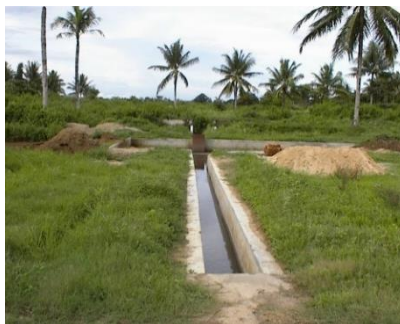
Figure 3.55: Effluent drain to settling ponds (Indonesia).
