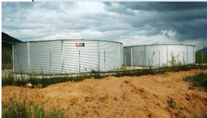
Figure 3.1: Water storage Tanks.
