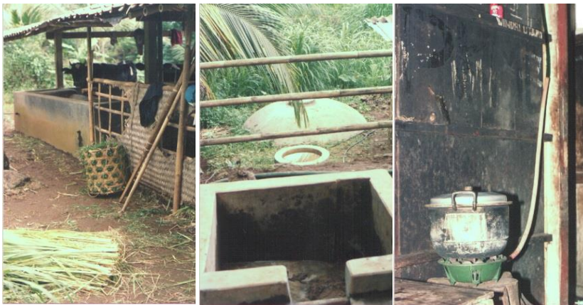
Figure 3.57: Cooking rice using methane from a biogas digester at a small holder dairy (Indonesia).
